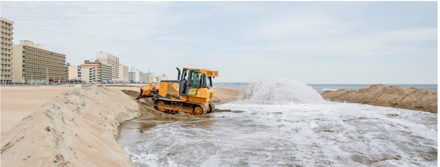
Beach nourishment in Virginia Beach, Virginia, where sand is dredged from offshore and placed along the shoreline to restore eroded beaches and strengthen coastal resilience. Projects like this have been carried out safely for decades under federal and state environmental oversight to protect communities, infrastructure, and public beaches. Photo Courtesy of City of Virginia Beach.
